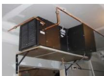
**A. Wine Guardian system must be mounted horizontally on its base as shown and be level to +/- 1/4" (0.6 cm) end to end and 1/8" (0.3 cm) side to side.**
