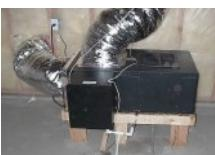
**B.** Mount unit in a location that is easily accessible for service and allow at least 3 feet (1 meter) for clearance on either side of the system for maintenance.
